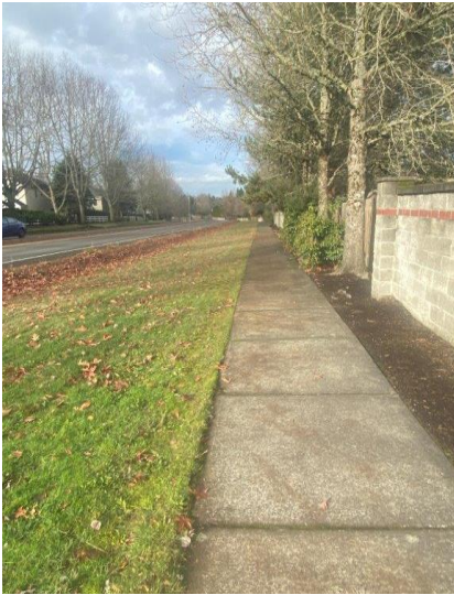
Concrete Safety Repair
