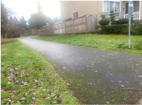
Paving Asphalt-Repair, Crackseal & Sealcoat
