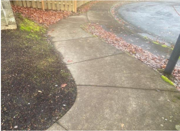
Concrete Safety Repair
