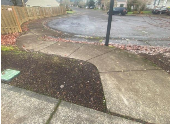
Concrete Safety Repair
